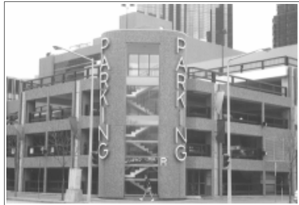
Parkade staircase allows natural light and natural surveillance.
