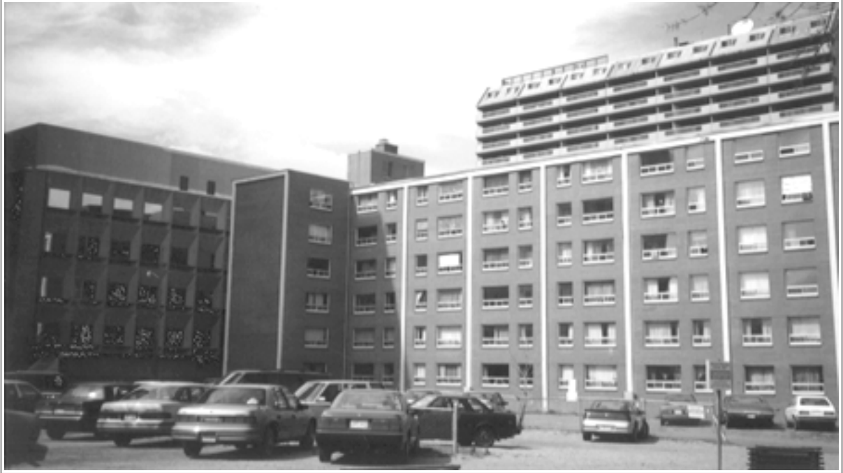
Parking area visible from nearby buildings.
