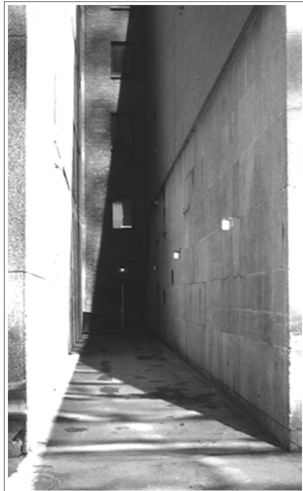
Deep recessed fire escape could act as an entrapment spot despite being lit.
