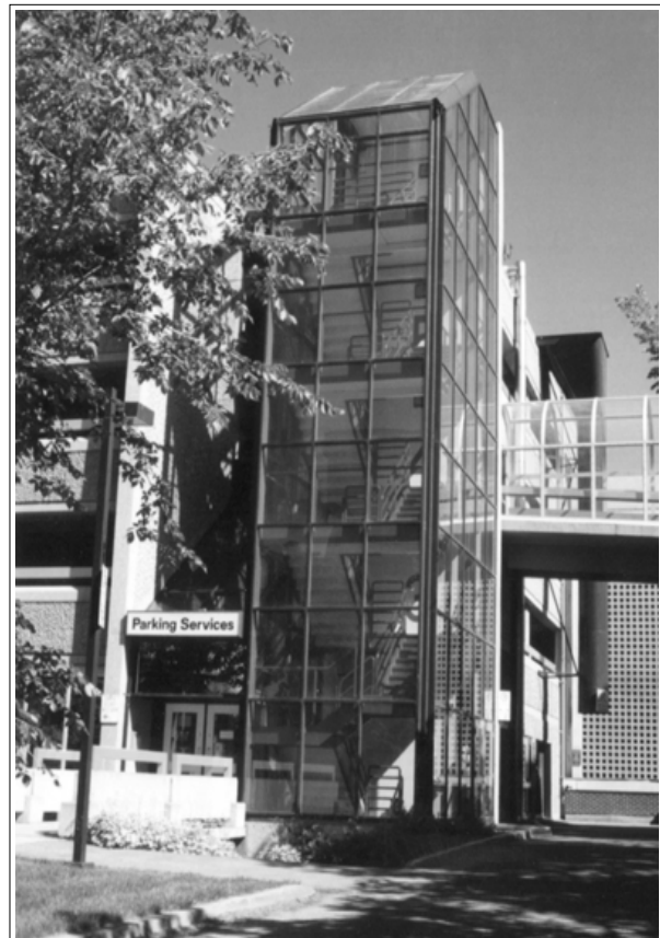
Glass enclosed stairwell design allows for clear sightlines and visibility.
