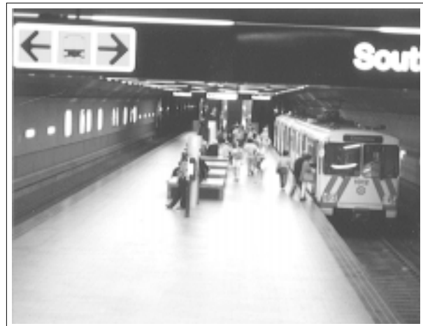
LRT stations provide HELP Telephones, good signs and visibility.
