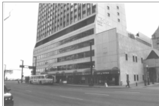
MacDonald Place provides a land use mix of retail, office and residential.
