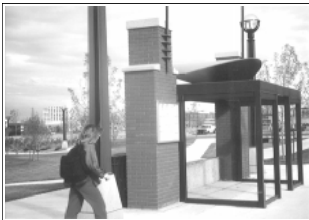
A special bus shelter design in downtown provides a wider exit to reduce the possibility of entrapment.
