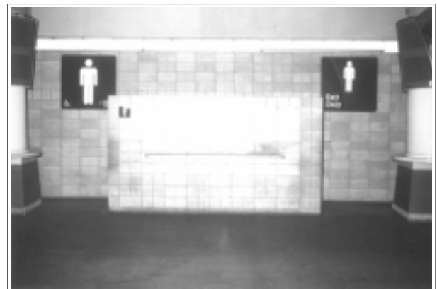
Washroom entry without doors reduces entrapment.
