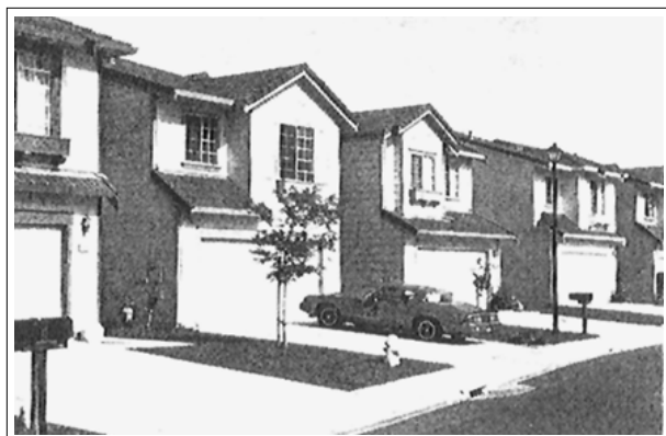
New houses (1980's) with double garages in front with family living facing backyard provides less street surveillance.
